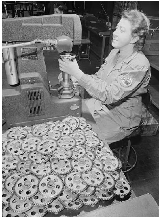
Magneto driving gears for Pratt & Whitney engines are tested for hardness (1942). Source: Library of Congress.
