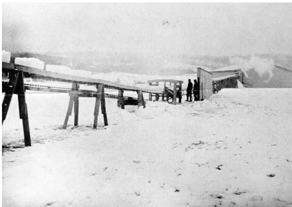
Another view of the conveyor belt / ice chute with blocks of ice moving towards Perry's ice house. ~1926. Courtesy of Joe Froehlich.
